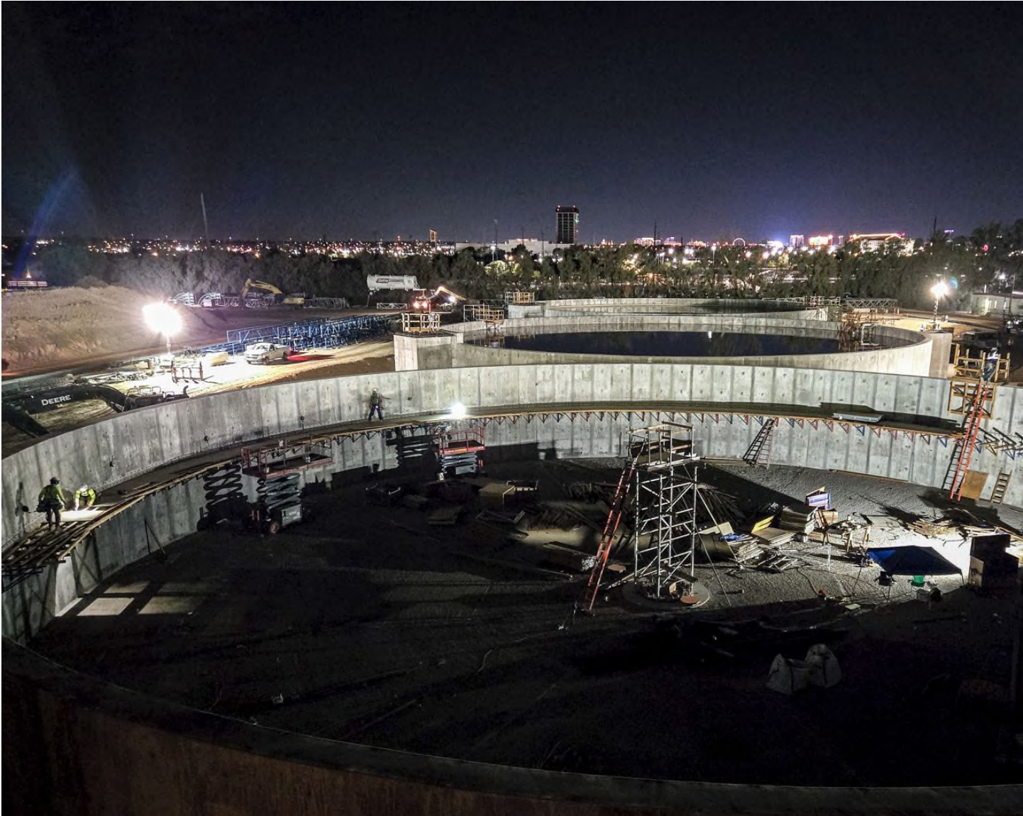
Construction continues through the night at the main Flamingo Plant
