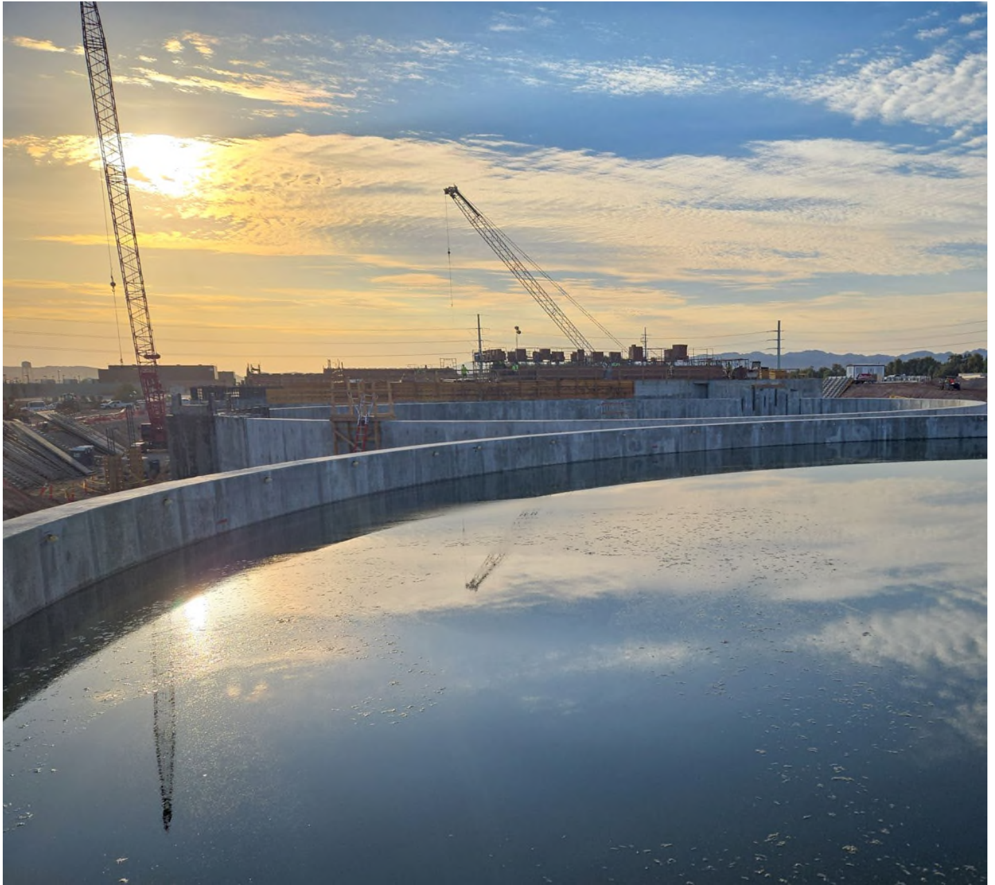
Water leak testing of a clarifier at the main Flamingo Plant
